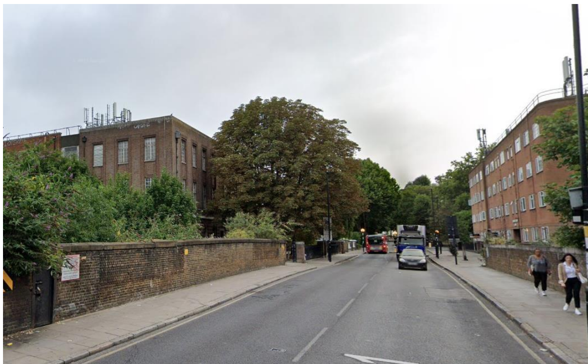
Image 3 – View of host building (left) from public highway of Highbury Grove, looking north
