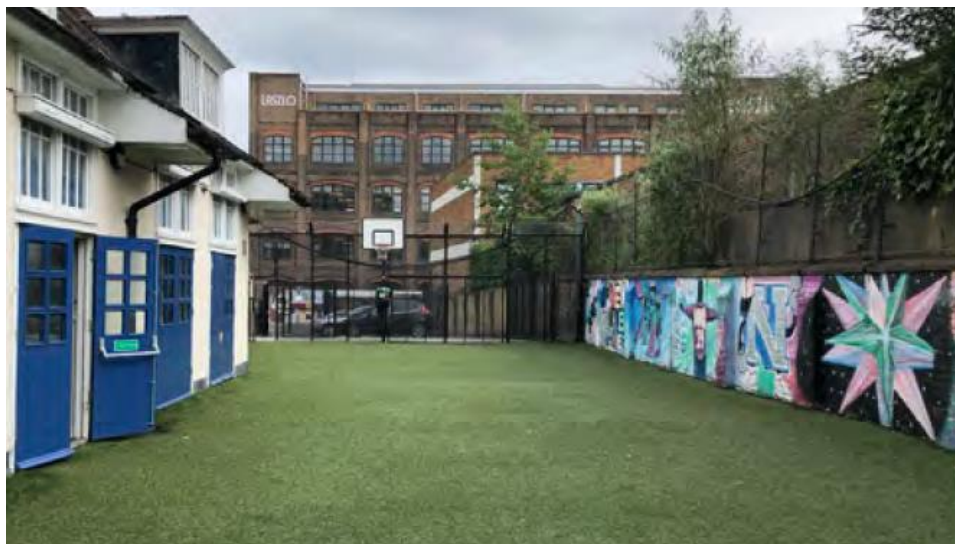
Figure 5 – View north-west to south-east (towards Elthorne Road)
