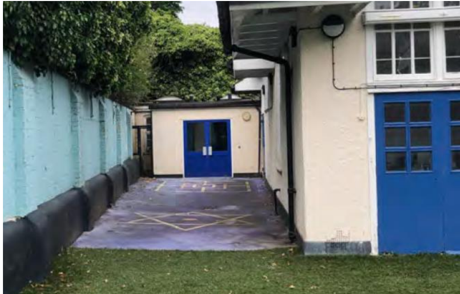
Figure 6 – View south-east to north-west (towards Giesbach Road)
