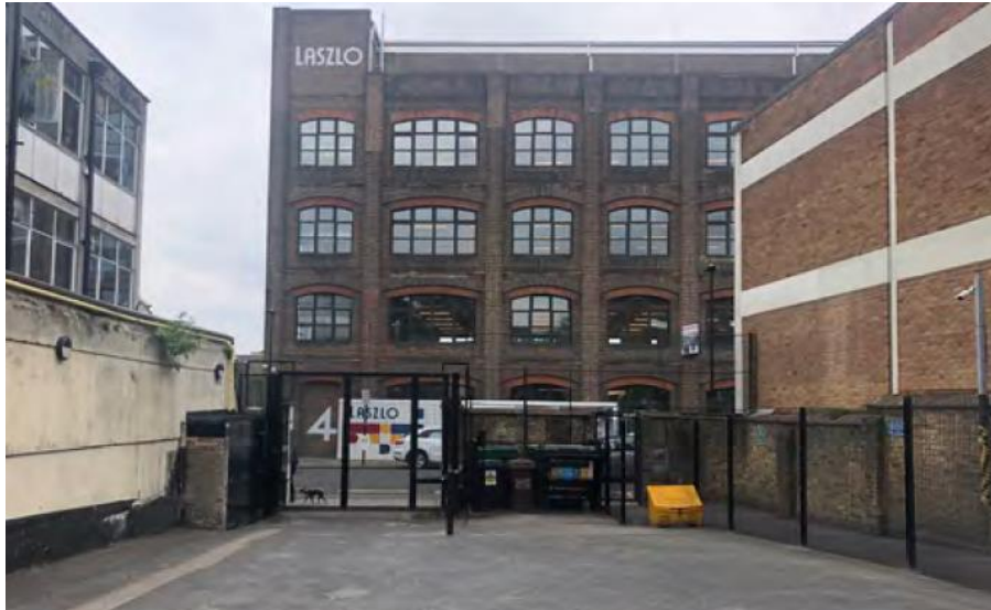
Figure 9 – View of existing concrete playground area (towards Elthorne Road)
